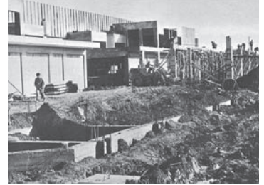
Formation of Kordsa Turkey Tire Cord Fabric Plant
